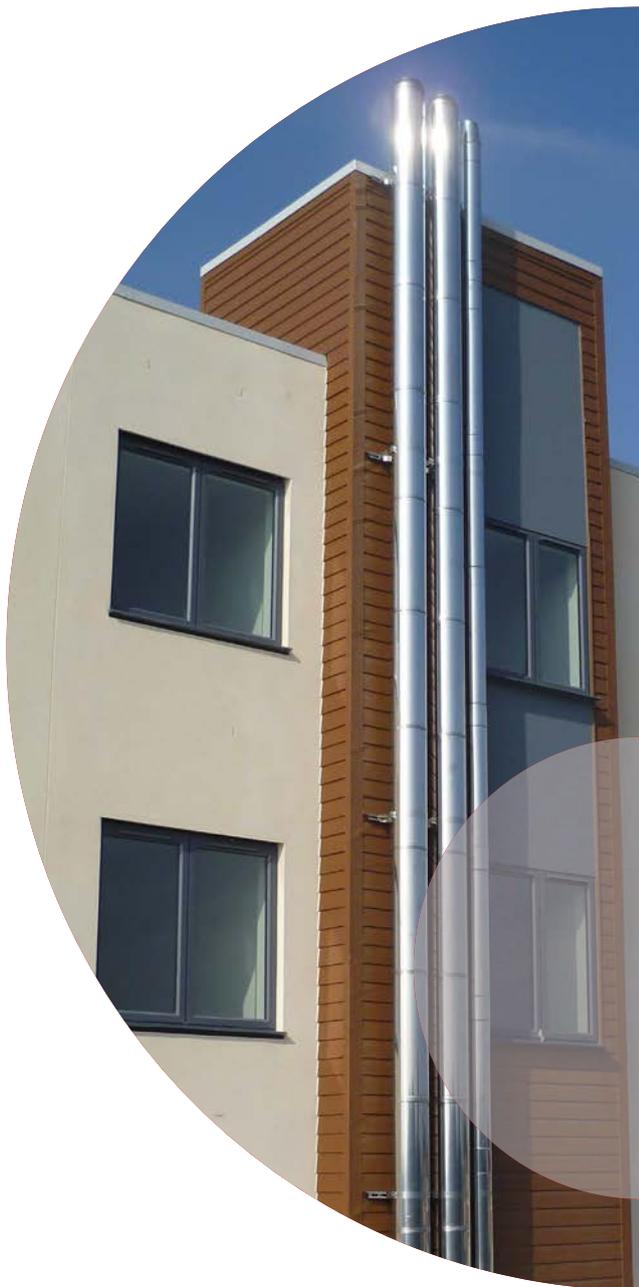
**SUPRA PLUS is British built** and specifically designed for today's modern high efficiency appliances that operate under positive pressure and condensing condition.
